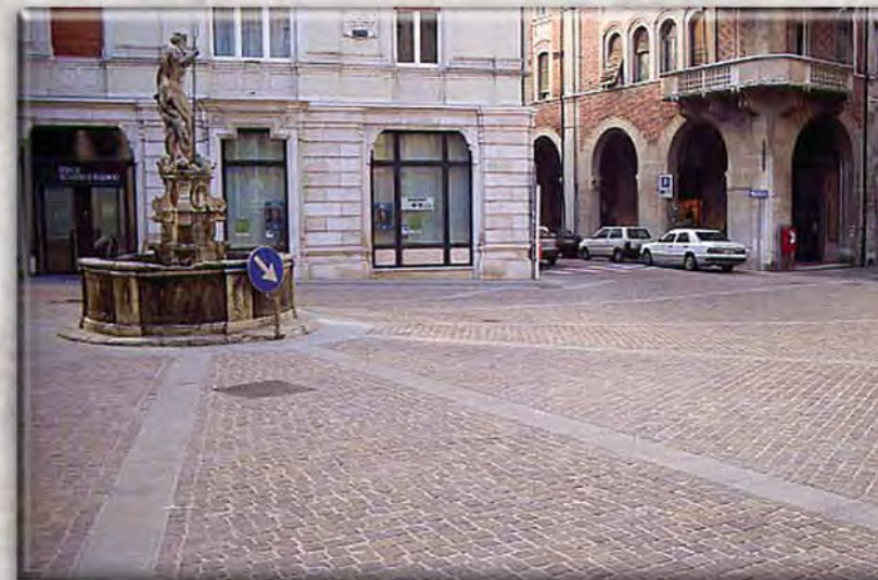
Granite cobble stone paved streets that were built hundreds of years ago are still being used in many parts of Europe
